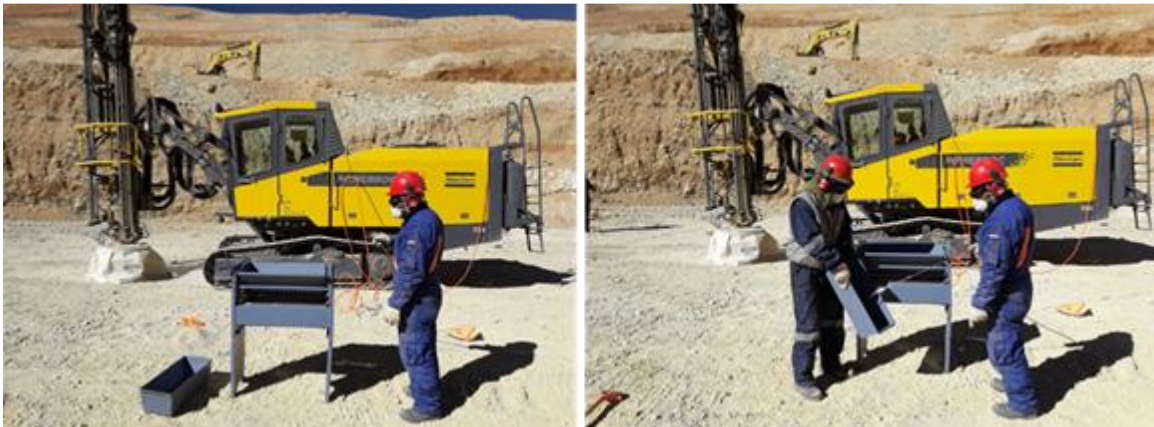
Figure 10.3: Drill Machine and Splitter
